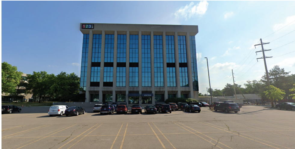
Figure 2 123Net Data Center 1 in Southfield
