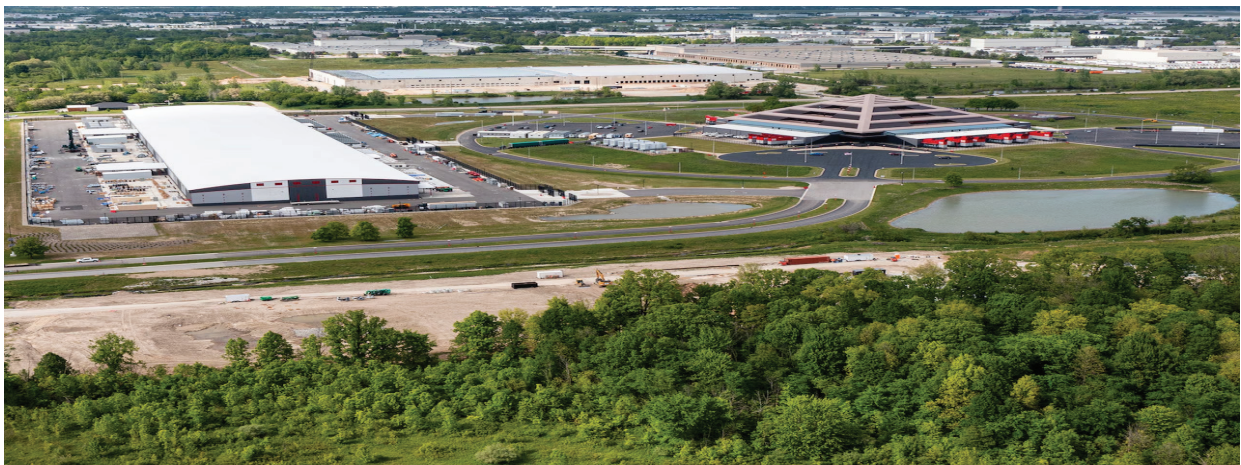
Figure 1 Switch 'The Pyramid' campus near Grand Rapids
