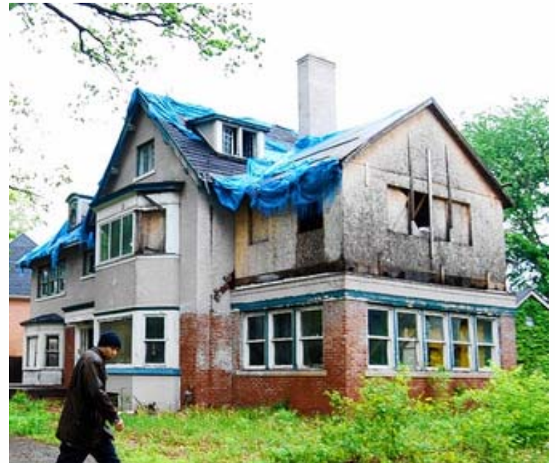
Mitt Romney's boyhood home prior to demolition
